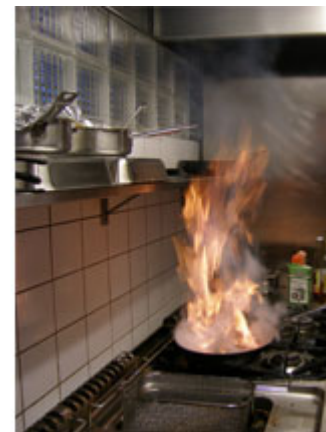
Without suppression, a stovetop fire may spread quickly into the vent system.
