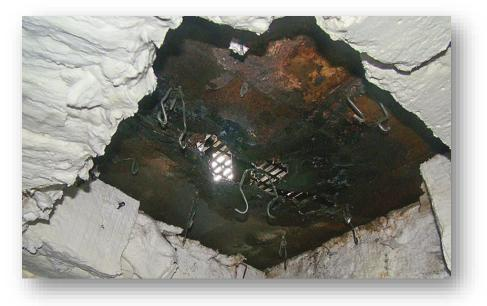
whether they were the root cause in the event of failure. Look for hot spots outside the unit. If the wall is in bad shape, this may indicate issues with the backup lining. To address voids, pump hot-spot repair materials in from the outside of an operating unit.
